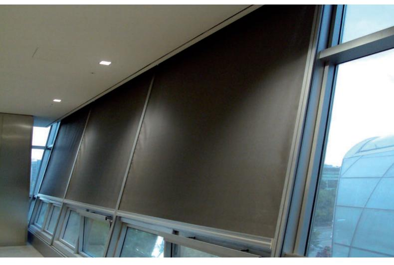
Somfy Korea installed guide-rail type roller screens to be used on inclined windows, applied to most parts of the building. To comply with the city's low energy plan, Somfy Korea suggested using animeo LON whose open protocol is capable of controlling motorized roller screens, HVAC and lighting.
