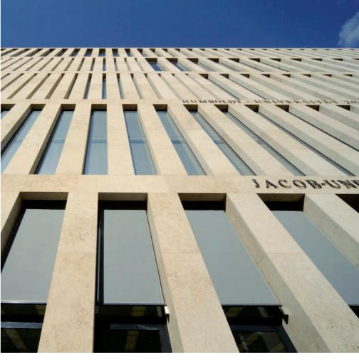
The Jacob und Wilhelm Grimm Zentrum is a building boasting cubist strictness and clarity. The deeply inset window openings have no frames or ledges, while their different sizes ensure architectural diversity. All openings are fitted with automatically-operated sunshades
