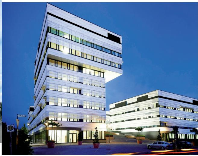
animeo IB+ was the only solution on the market to satisfy the requirements for handling the shutters in terms of specific weather conditions. Three protection functions were implemented – wind protection, snow and ice protection and a security function. High wind loads start the wind protection function: the shutters close.
